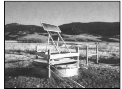
A solar-powered pump and stock tank are keeping cattle out of streams.
