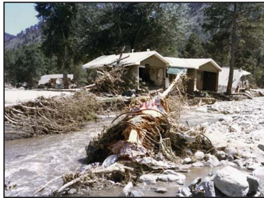
Cedar Cove, situated just above the narrows in the Big Thompson Canyon, was hard hit by the flood.
